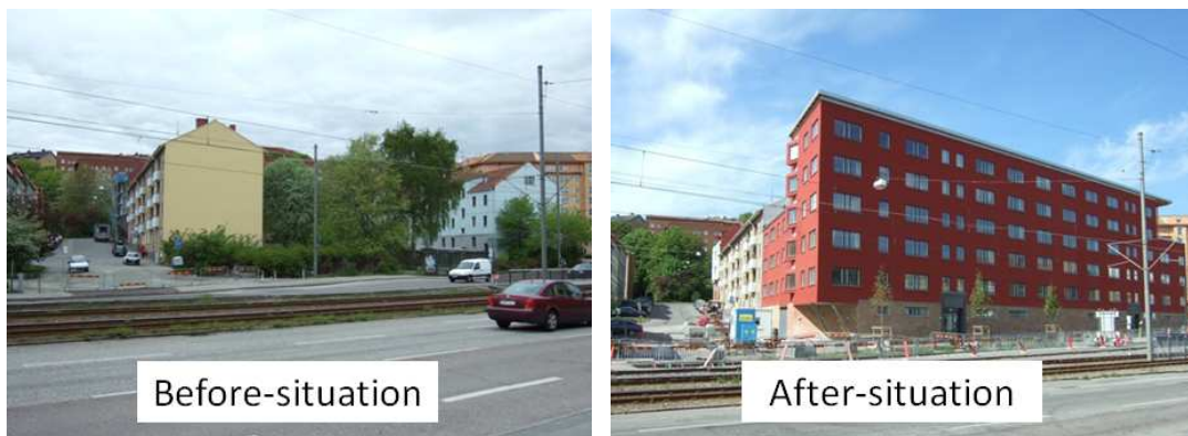
Figure 2.8. Pictures of the situations before and after the intervention in Gothenburg (Bomgatan). The picture on the left shows the area in 2006 with the open courtyard facing a busy road. The picture on the right (2009) shows the new building that fills the previous gap.
