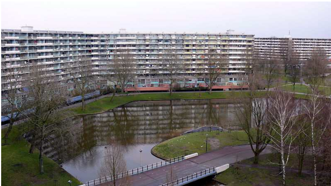
Figure 3. View of the Amsterdam quarter Bijlmermeer built in the 1970s (picture 2008).
